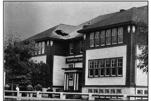
Courtenay Elementary - Exterior
