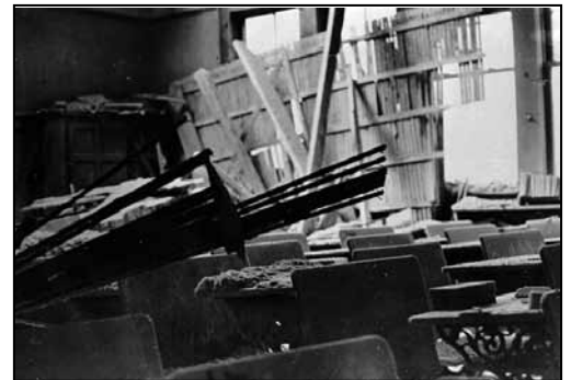
Courtenay Elementary - Interior
